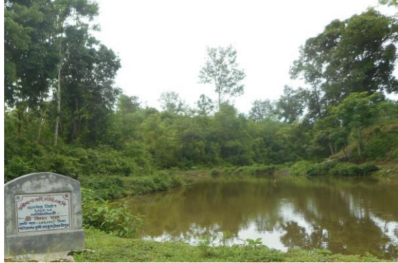
Construction of Farm Pond of Shri Bimal Das
