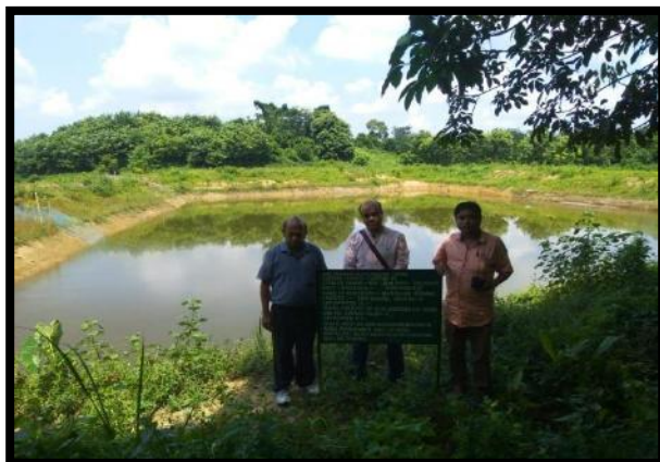
Construction of Farm Pond of Sri Bishnu Dev Barma
