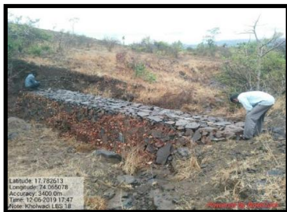
MEASUREMENTS OF THE LOOSE BOLDER STRUCTURE BEING TAKEN
