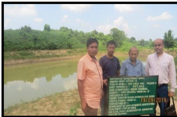
Construction of Farm Pond of Sri Bishnu Debbarma
