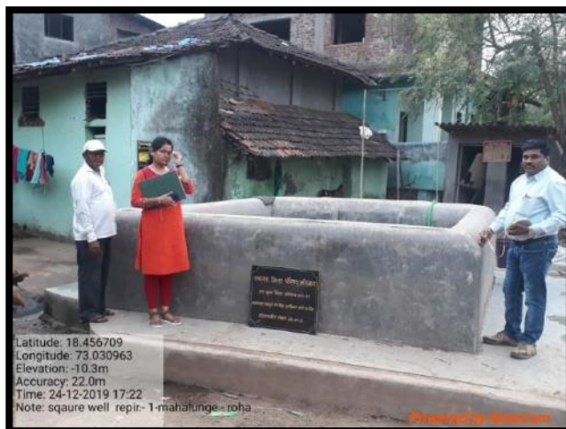
WELL REPAIR IN RAIGARH, MAHARASHTRA UNDER THE MJSA
