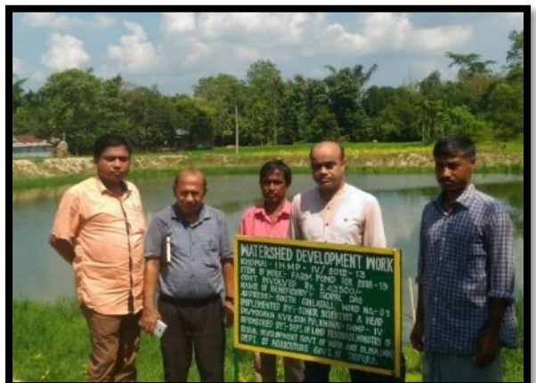
Construction of Farm Pond of Shri Gopal Das
