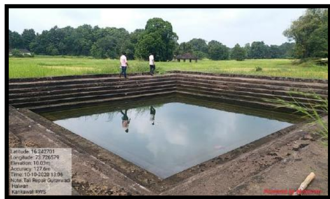
POND REPAIR UNDER THE MJSA
