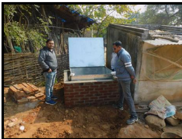
INSTALLATION OF LOW COST COOLING CHAMBER
