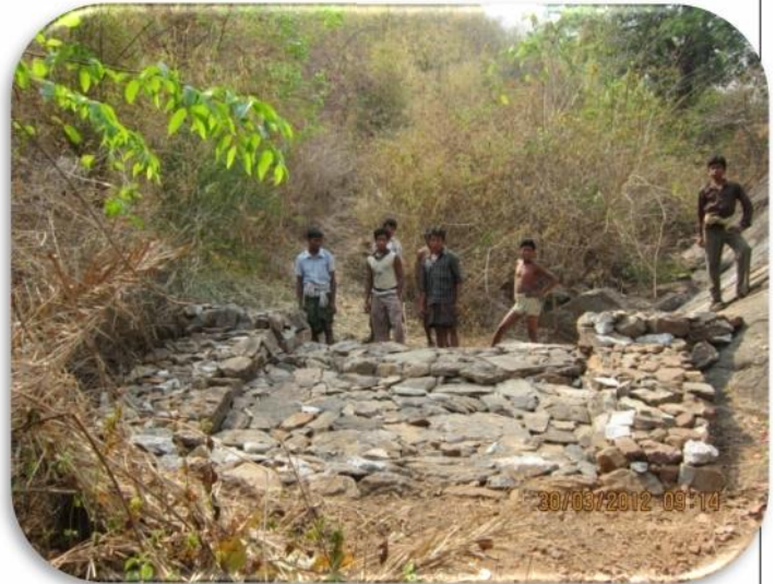
Drainage Line treatment with stone works
