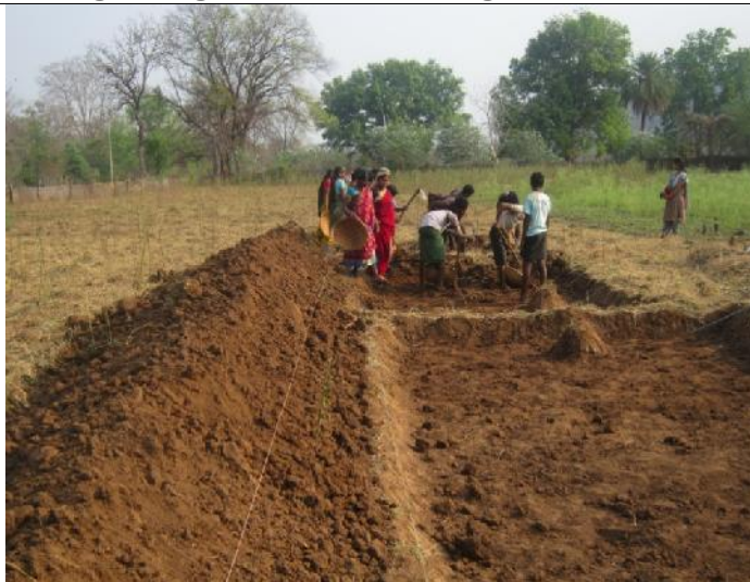
Soil works before WADI plantation
