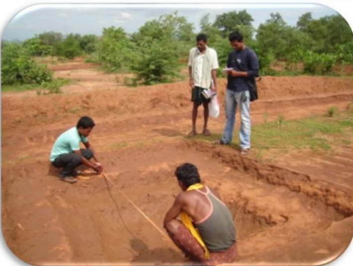
Measurement of completed works
