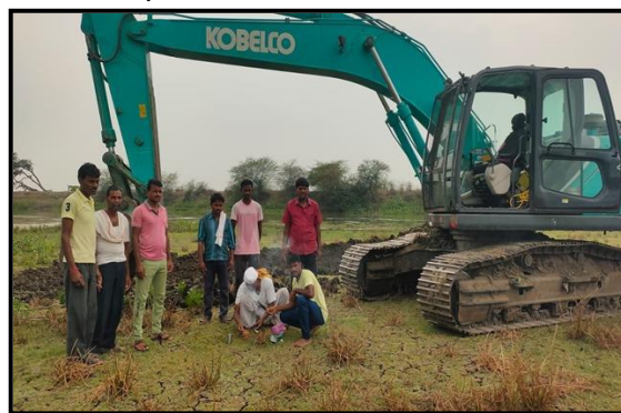
Work inauguration by community
